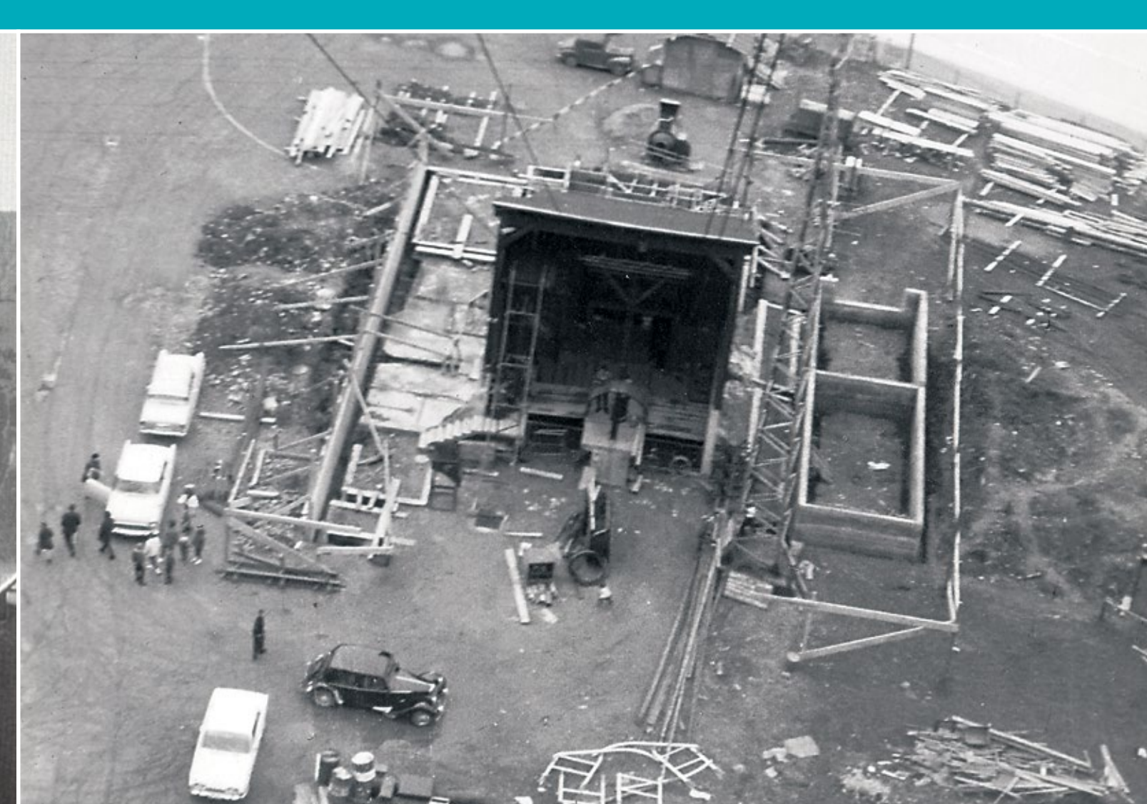
Cablecar bottom station under construction 1954-5 10
