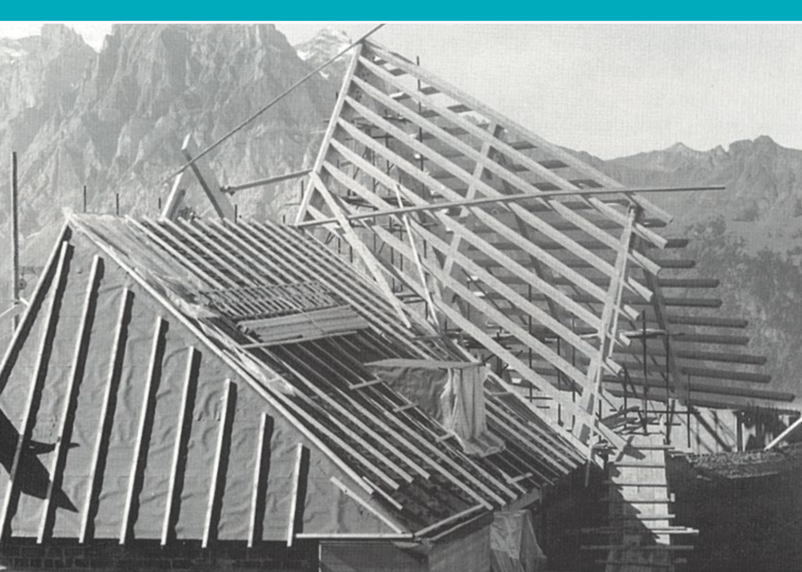
1968 Marien-Chapel under construction 10
