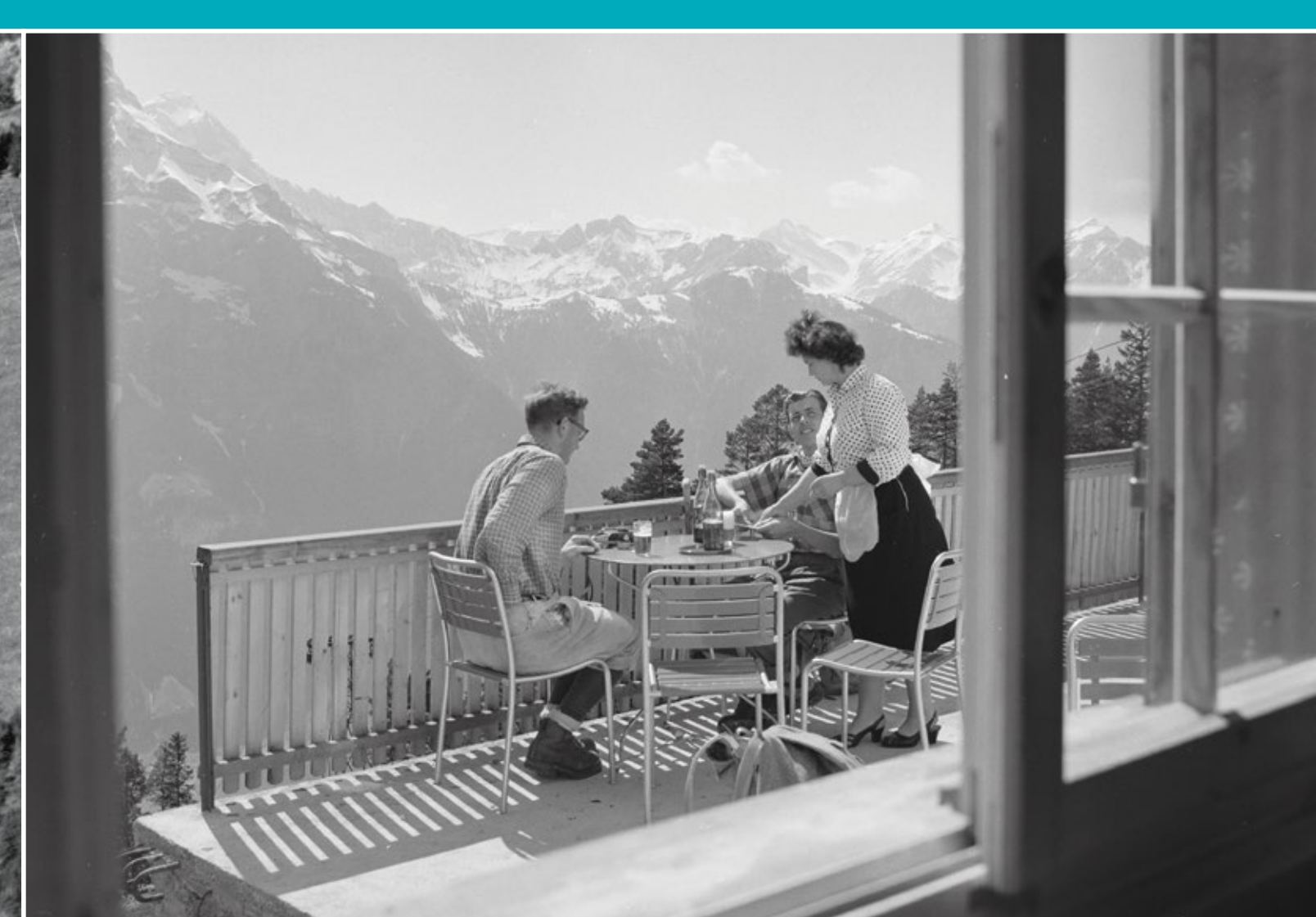
First guests enjoying the restaurant terrace (notice the unfinished terrace construction!) 10
