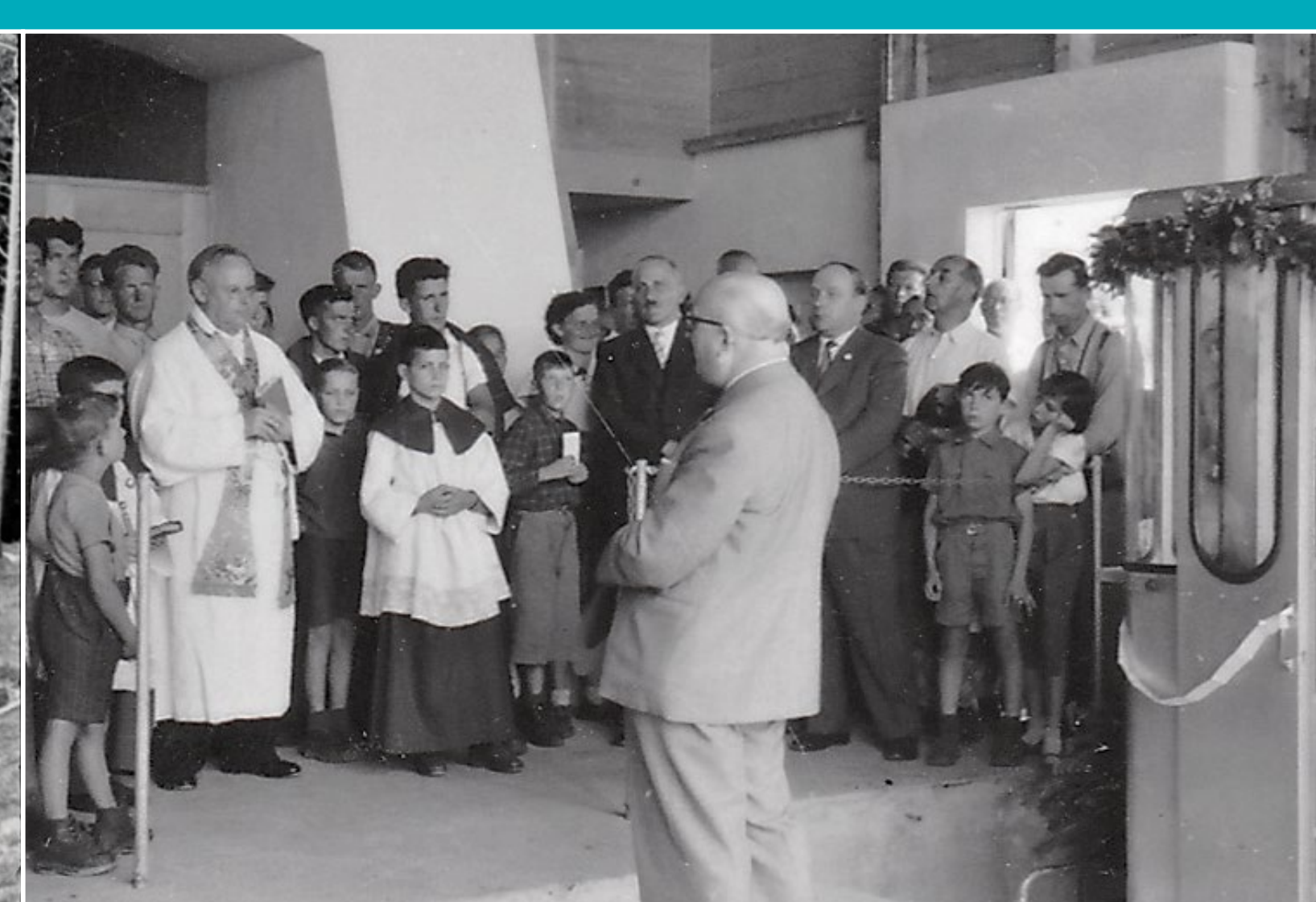
Opening ceremony of the cable car, at the mountain station, 1955 10
